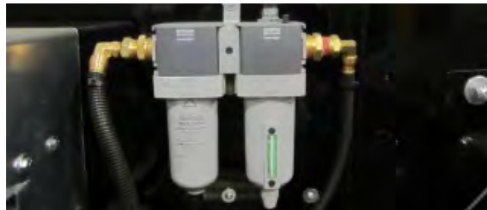
Figure 1: Air Filter And Lubricator
